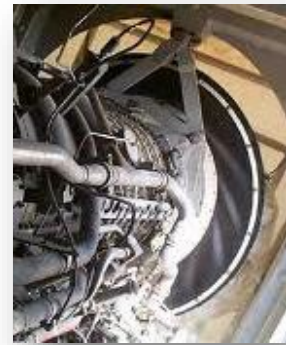
GAS TURBINE BARRIER WALL GASKET PN: CAP-3471-1
